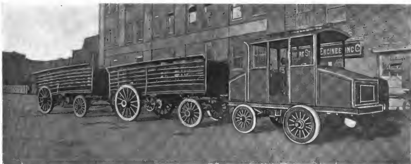
Fig. 5.—Another example of the same type of gasoline-electric road train made by the Gibbs Engineering Company.
